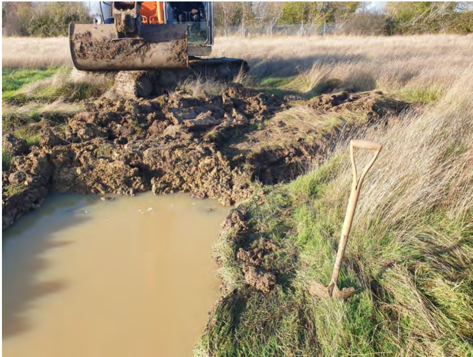
Plate 1 Working shot of the excavator being used to bail out flooded trenches to allow hand excavation of features. A frequent occurrence due to heavy rainfall
